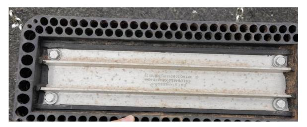
During the weekly inspections the flat swing fixtures that connect the chain to the seat are regularly tightened as the screws are old and have been cross threaded.
